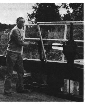
CLOSING the "paddle" (valve) of a lock gate.
